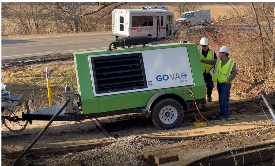
Figure 6. Some evacuation sites can involve difficult access.
