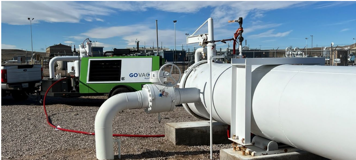
Figure 11. Pigging operation on a 36-inch pipeline.
